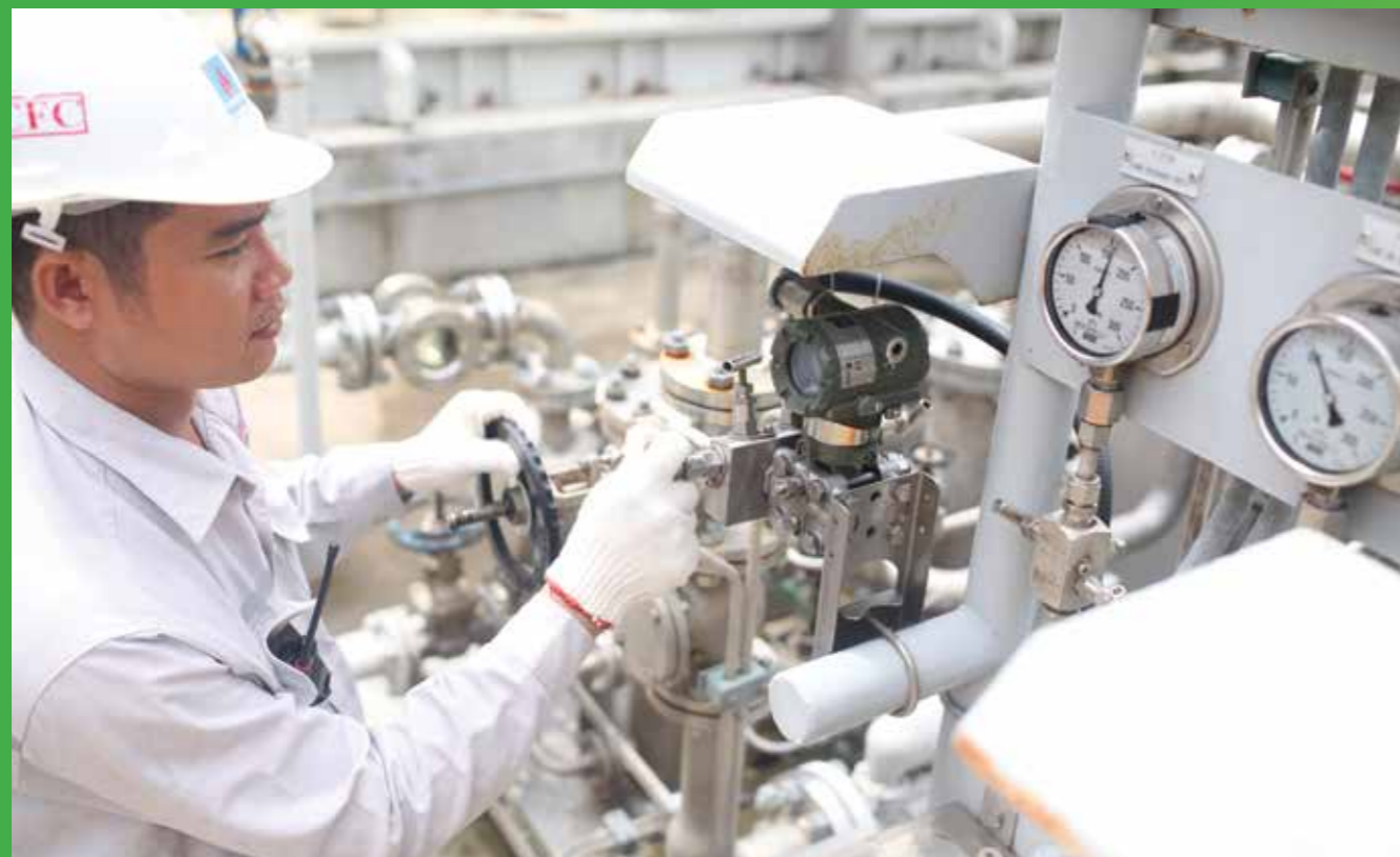
Periodically maintenance at the Ca Mau Fertilizer plant
